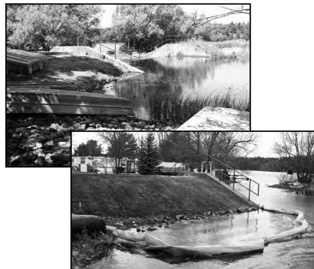
These photos show the erosion adjacent to the dam before and after the regrading and erosion control work was completed.
