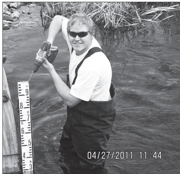
St. Lawrence College student Jon Donaher installs a staff gauge at Temperance Lake. These gauges help CRCA measure water levels on the lakes.
